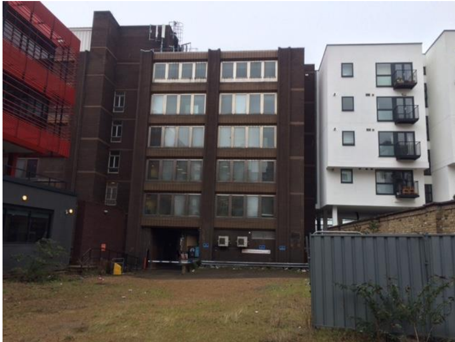
Image 2 – View from the site towards 6-storey office building fronting Turnmill Street.
