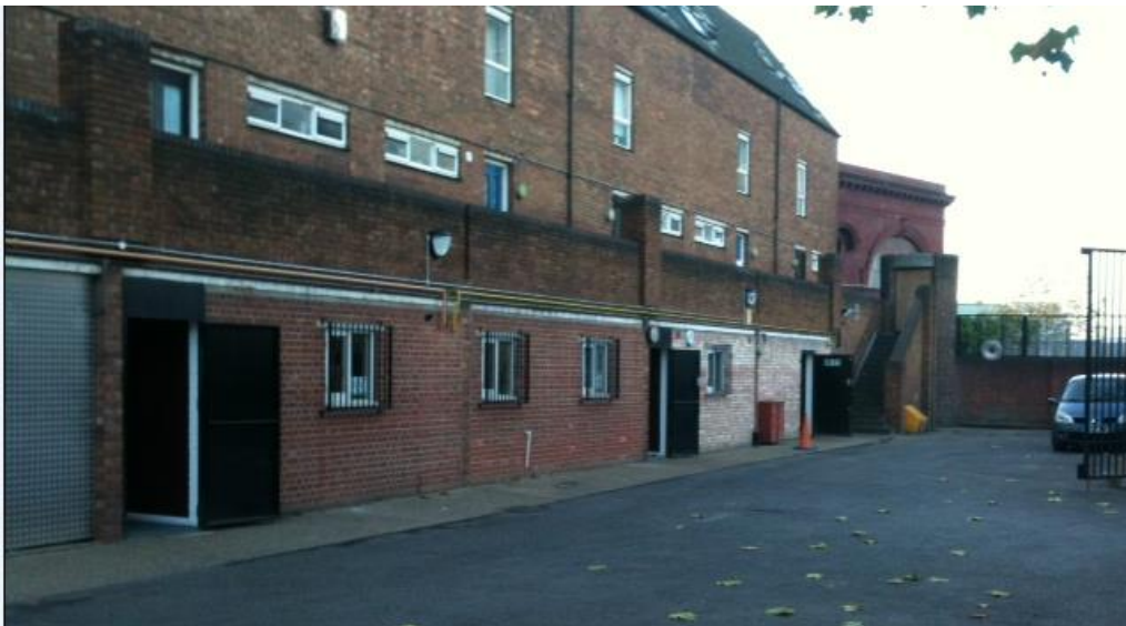
Photo 1: View of office space (previous undercroft)
