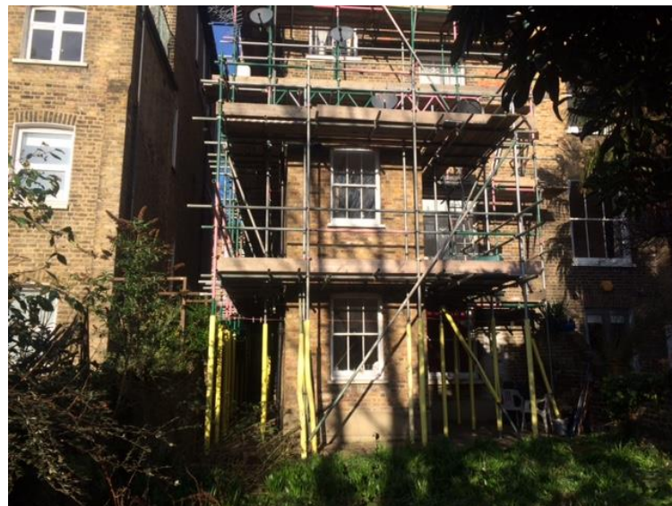
Rear elevation of the semi-detached building
