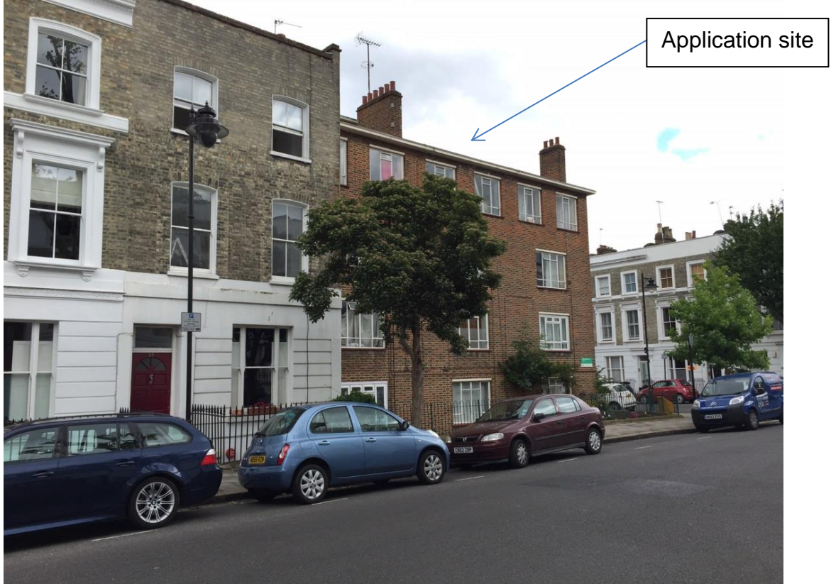
IMAGE 1: The west elevation of the building fronting Florence Street
