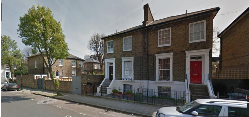
Image 4 – View of rear elevation at 1 Halliford Street
