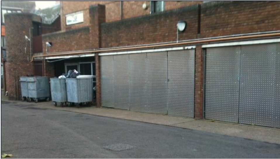
Photo 2: View of storage space (previous undercroft)
