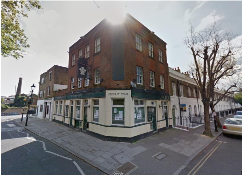
Image 2: View of frontage of building from Vincent Terrace
