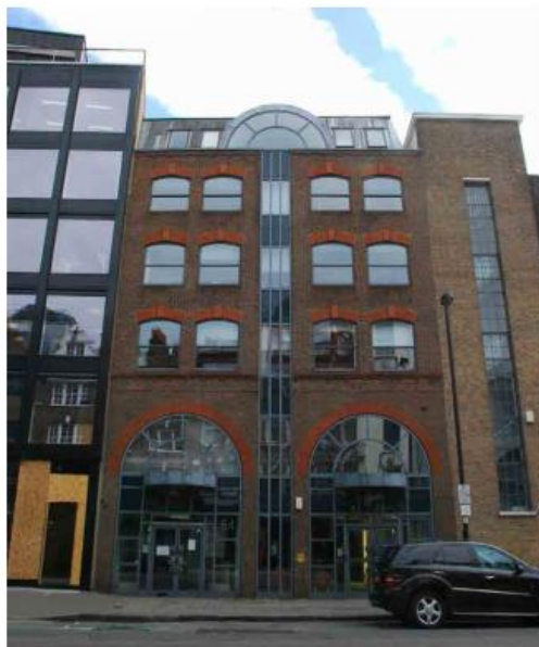
Image 1: Front Elevation of the application site
